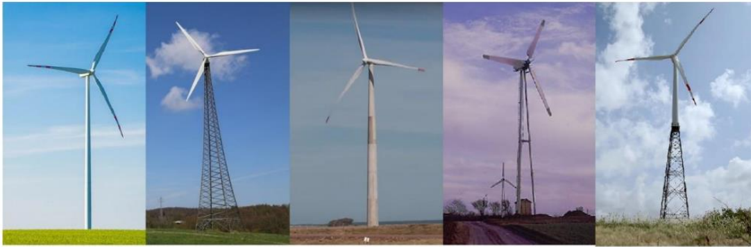
Types of wind turbine towers [1]
