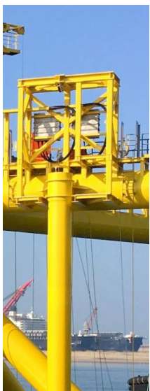
Disconnectable Dry Spliced Connection (Principal Power)
